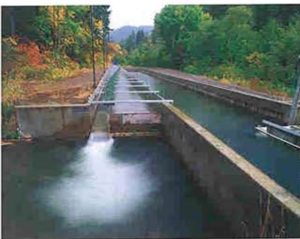
A Farmers Screen test site on an 85-cfs diversion on the Hood River in Oregon.
