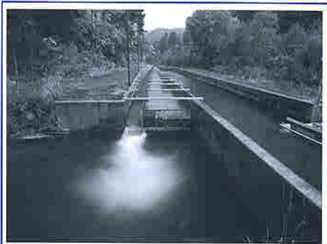
Figure 1. The Farmers Screen in Operation, Farmers Irrigation District's Davenport Screen (80 cfs) was the first installation installed in 2002.
