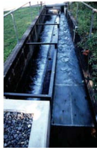
The Farmers Screen utilizes the dynamics of water movement to screen water while safely sweeping fish and debris back to the river or stream.
