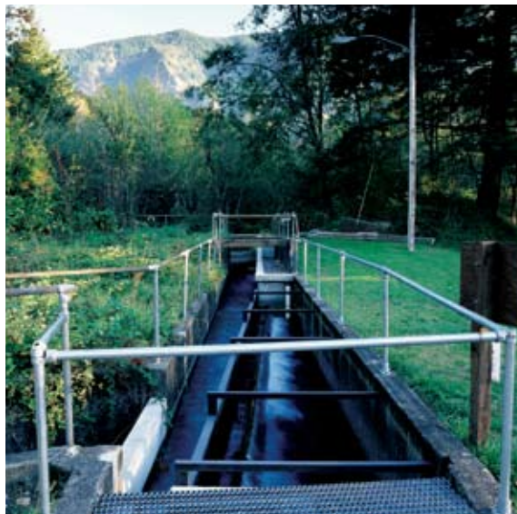
The Farmers Screen utilizes the dynamics of water movement to screen water while safely sweeping fish and debris back to the river or stream.
